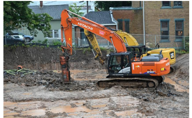
Excavation & rock breaking for foundations
