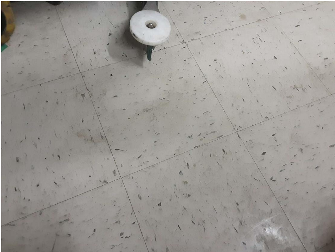
S0009C (Confirmed Asbestos), 12" white with blue flecks, Floor, Vinyl Floor Tile and Mastic, Custodian Room (Location #: 1)
