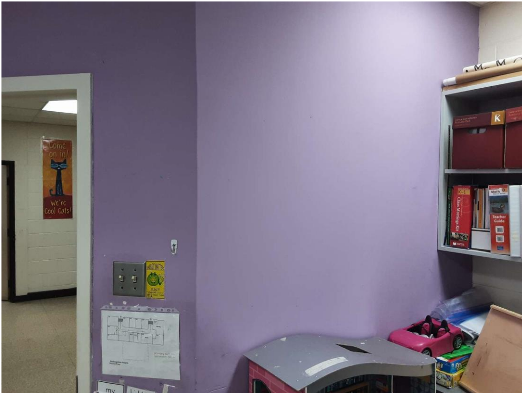
V9500 (Presumed Lead), Purple, Wall, Classroom (Location #: 53) No discreet place to sample
