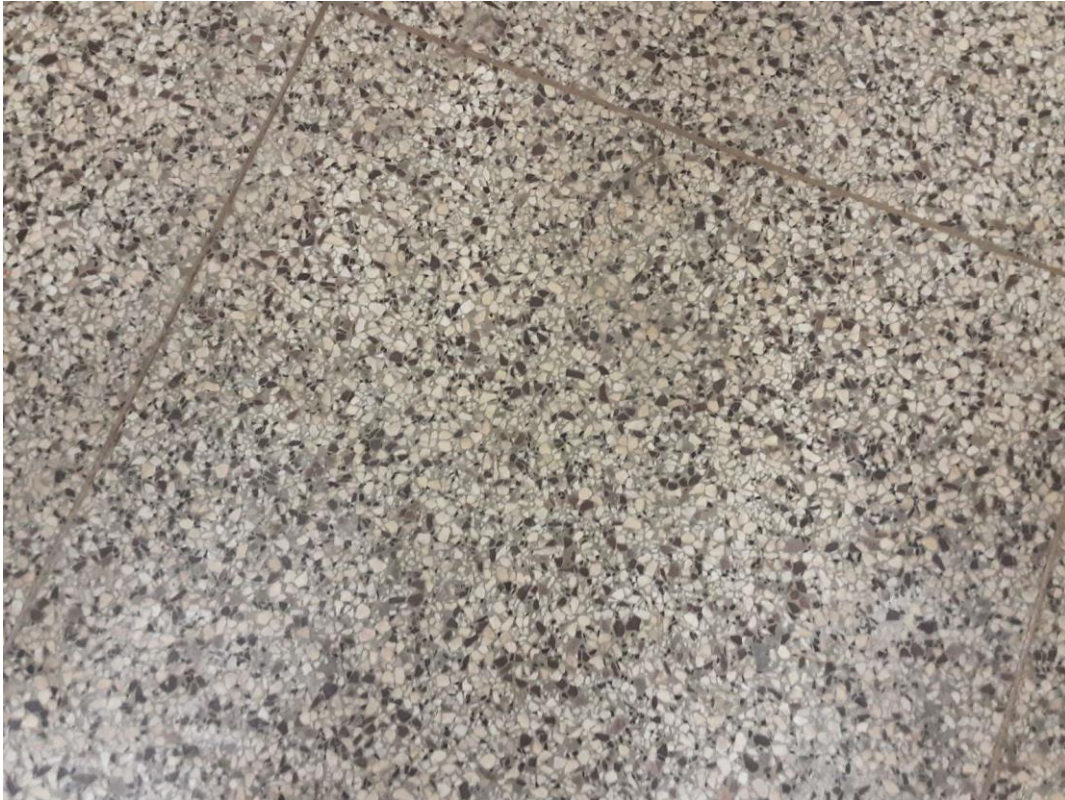
V9500 (Presumed Asbestos), Pebble pattern, Floor, Terrazzo, Washroom (Location #: 2)
