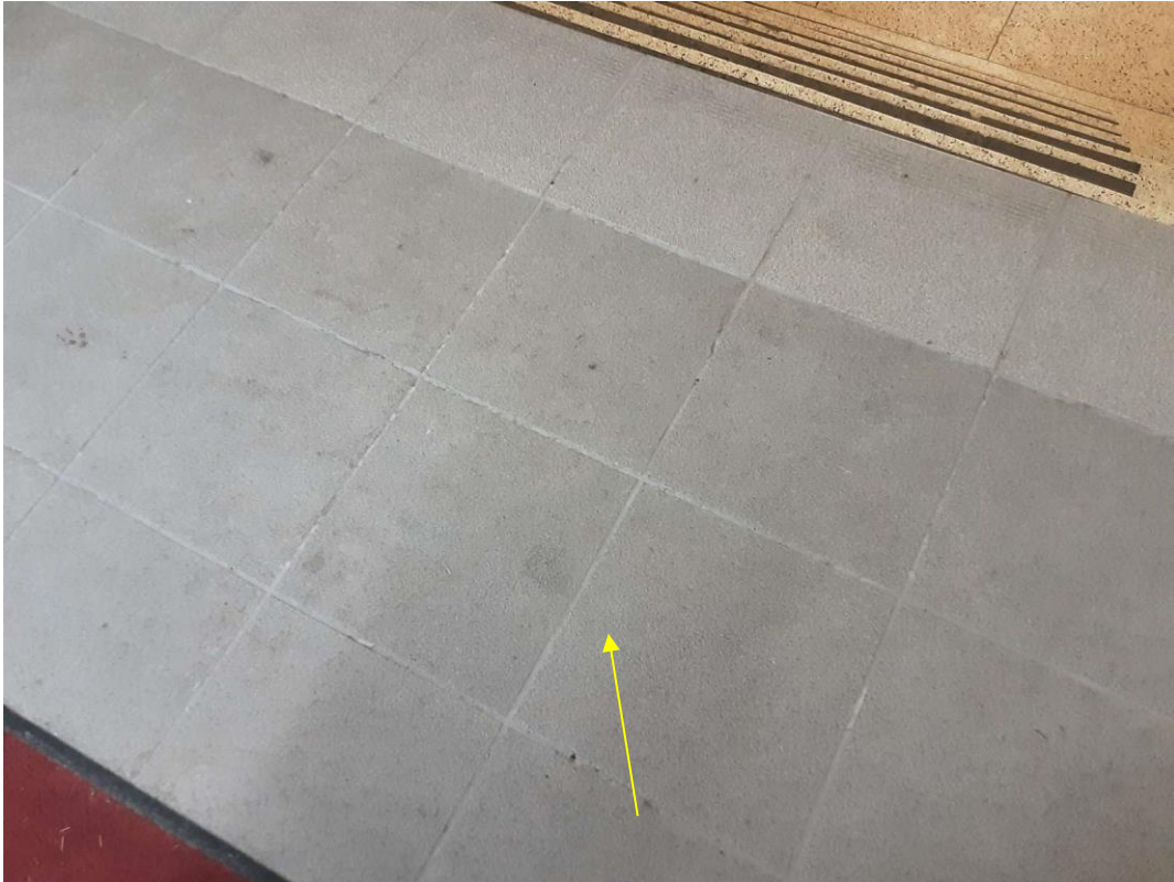
V9500 (Presumed Asbestos), 12" grey tiles, Floor, Thin-set under ceramic tiles, Stairwell (Location #: 67)
