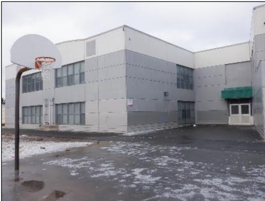
Photo 4 - General view of the south elevation, western portion.
