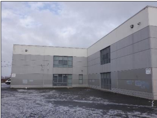
Photo 5 - General view of the west elevation, southern portion.
