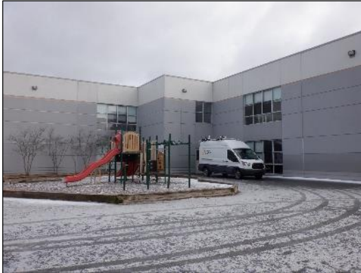
Photo 6 - General view of the west elevation, northern portion.
